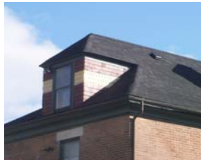
Deteriorated shingles & wood trim removed, replaced with new in same pattern & painted.
